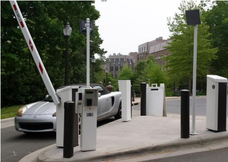
T2 Systems integrate with TagMaster NA solutions to optimize Duke University parking
